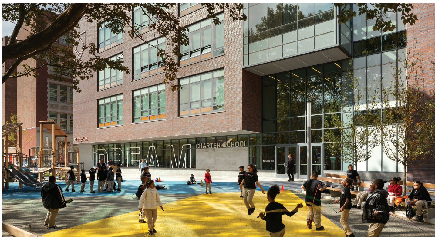
DREAM scholars enjoy recess outside their new school building in the renovated Blake Hobbes Park.
